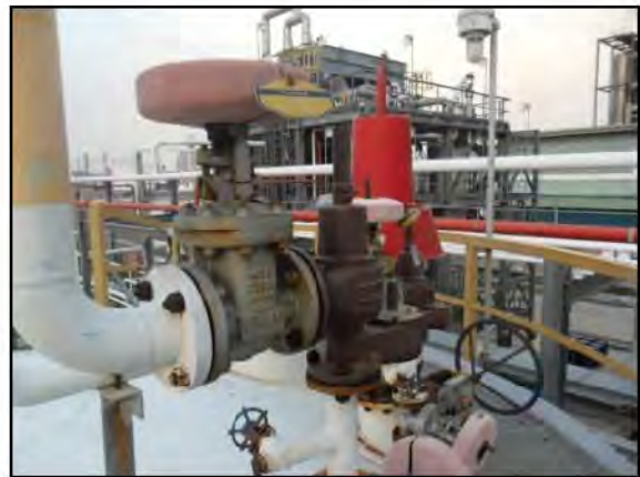
Pressure Vacuum Relief Valve
